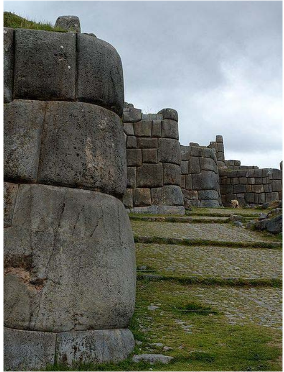
Sideways view of the walls of Sacsayhuamán showing the details of the stonework and the angle of the walls.
