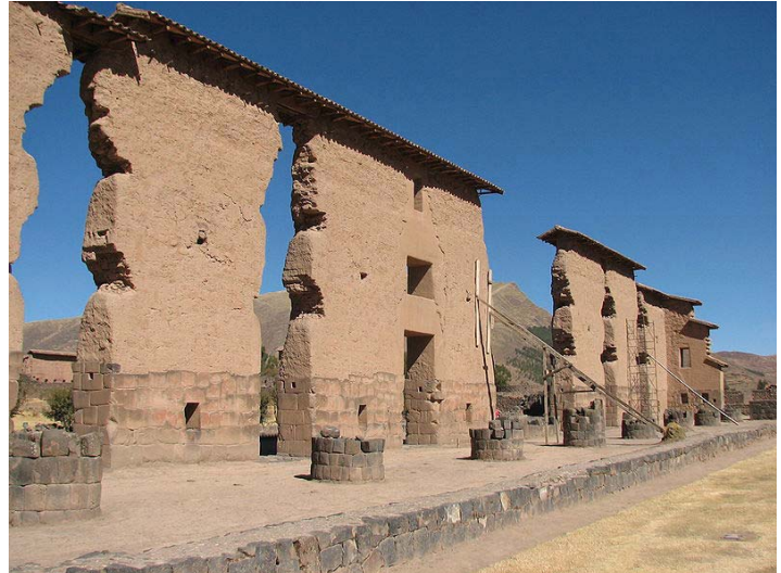
The central wall
